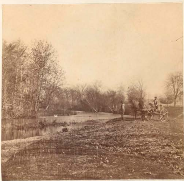
View of the Washaway - near Atherton Bridge.
